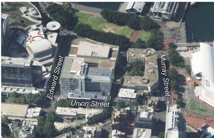
Figure 26 – oblique aerial of 2 Edward Street & 60 Union Street
